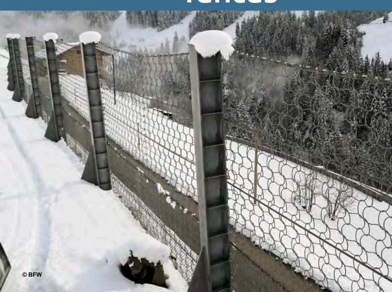
Snow catchment fences such as the SNOW-CATCHER do not prevent the initiation of avalanches but instead interact with an avalanche in the run-out or deposition zones in order to slow the avalanche and bring it to a standstill. This shortens the destructive reach of avalanches.
