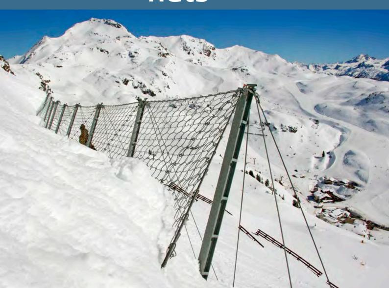
Snow nets prevent the development of avalanches by giving structural support to the snow mass in initiation zones having medium to large snow depths. This is in contrast to other approaches such as artificial release methods - e.g. by means of explosives - that initiate smaller avalanches before the hazard grows to an unmanageable size.
