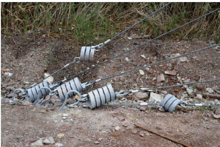
Brake elements are only found at the extremities of a system, directly at anchor points. All brake elements are connected with shackles to the ropes and can be easily changed. In this example, brake elements consist of large steel coils that unwind during impact.
