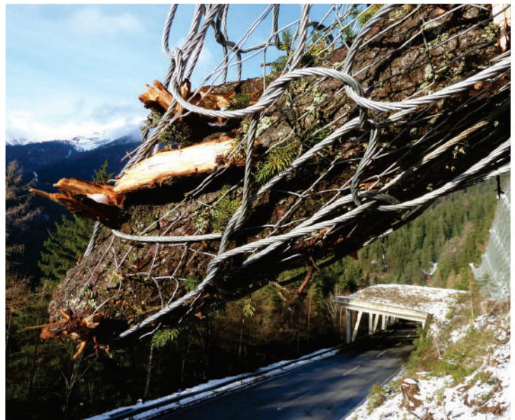
An example of a tree stem impact on a rockfall catchment fence.
