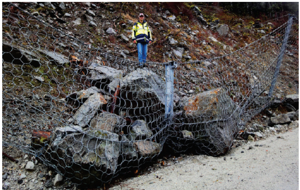
Two examples of hinged rockfall catchment fences impacted at and surrounding a post. Posts by Trumer are robust and can withstand direct impacts without compromising the systems integrity.
